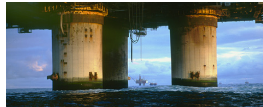
Statfjord platform NW of Bergen
